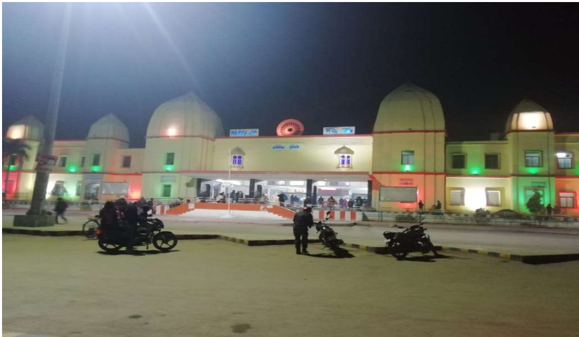
Fascad Lighting AT Mau Station
