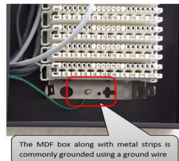
2. Insert the IPM in the Krone Module and it is mandatory to ground the IPM from its ground pin using a metal strip in the MDF.
