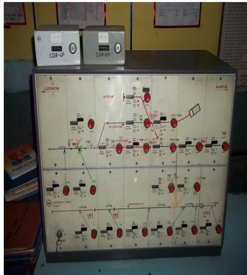
Multi Section Digital Axle Counter
