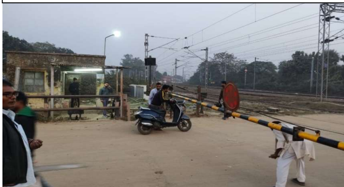
L C Gate with Electrically Operated Lifting Barrier with Sliding Boom
