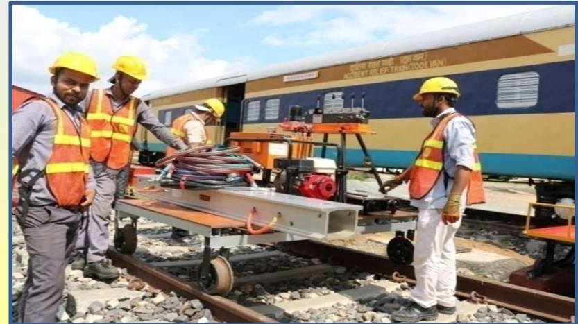
2. Local made 4 rail trolley for material movement
