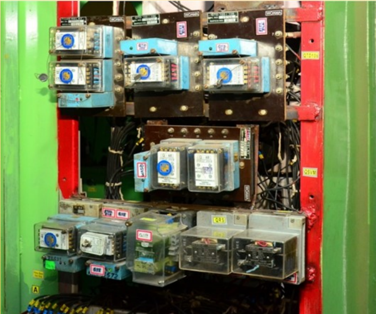
Relay Panel for displaying various types and modes of operation
